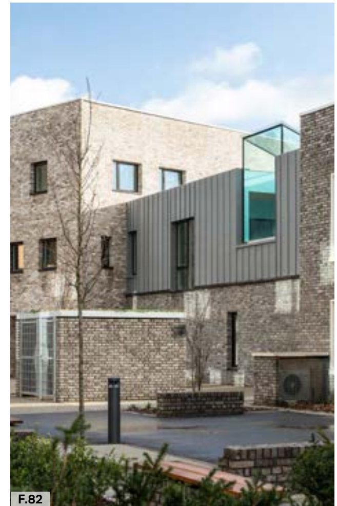
Figure 82: Refuse and heat pumps contextually screened by using the same materials used on the façade of buildings ( Image: TOWN, David Butler )
