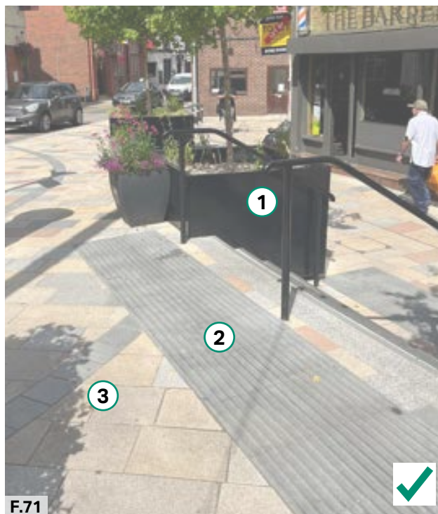
Figure 71: Change in level along Bridge Street made accessible with tactile paving and railings 1. Railings to assist users in moving between different levels in the street 2. Tactile paving to alert users of a change in level 3. High-quality surfacing referencing the hues of the streetscapes historic buildings
