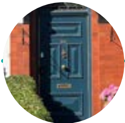
Timber panelled door
