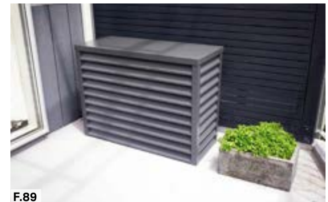
Figure 89: Air source heat pump housing covers the unit and harmonises with the building aesthetic
