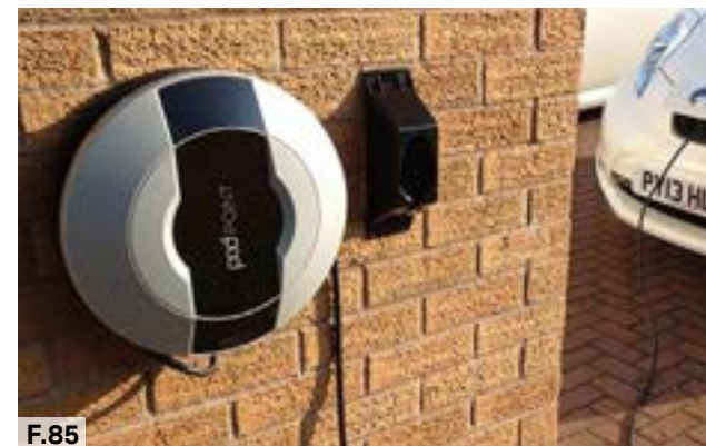
Figure 85: Home EV charging point hidden out of view at the rear / side elevation of a building
