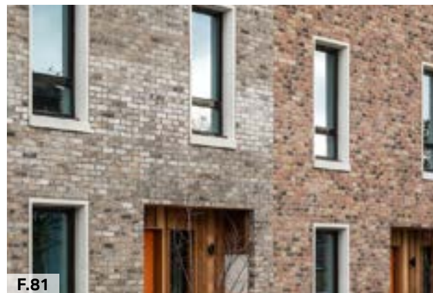
Figure 81: High-quality materials used on façades, within window / window frames, and doorways ( Image: TOWN, David Butler )
