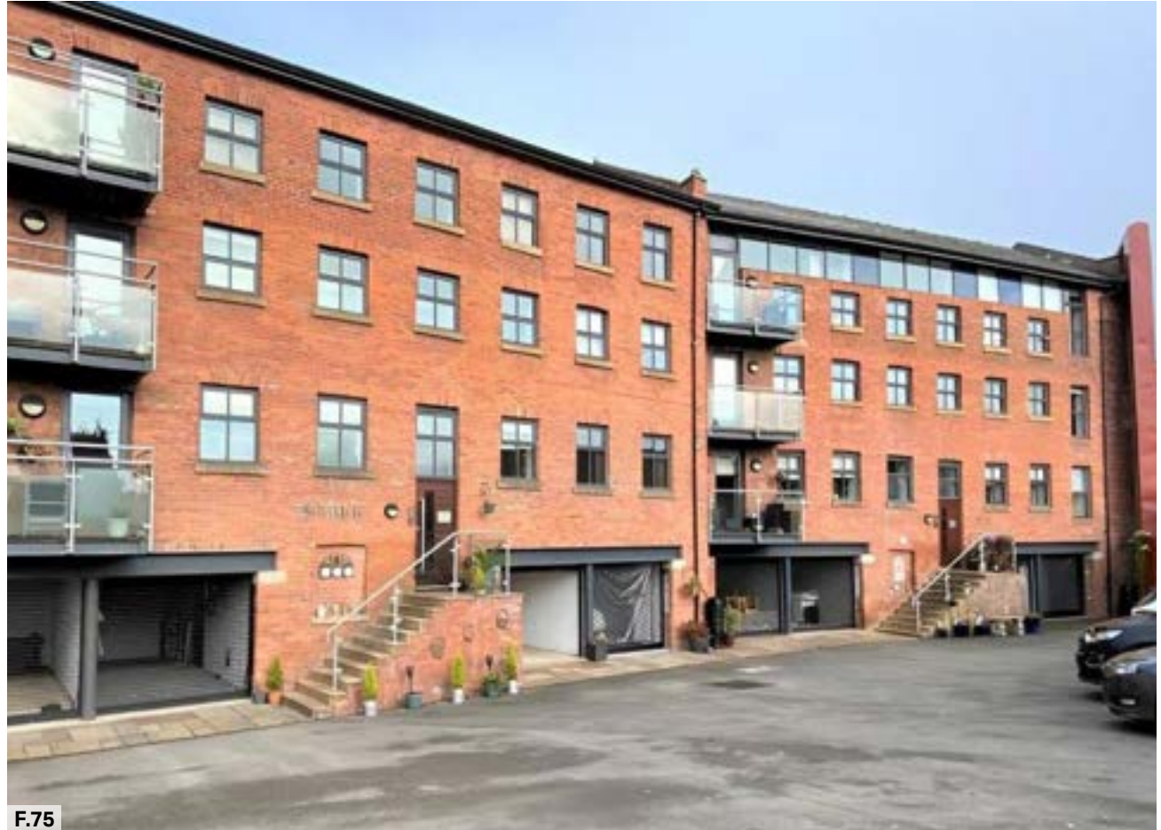
Figure 75: The Silk Mills - historic mill sensitively converted into a residential apartment building with balconies, new windows, and undercroft parking provided for residents
