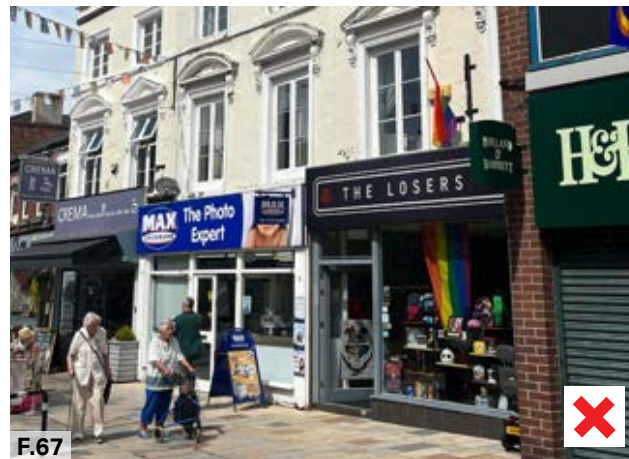
Figure 67: Imposing and nondescript frontages degrade the character of the historic streetscape
